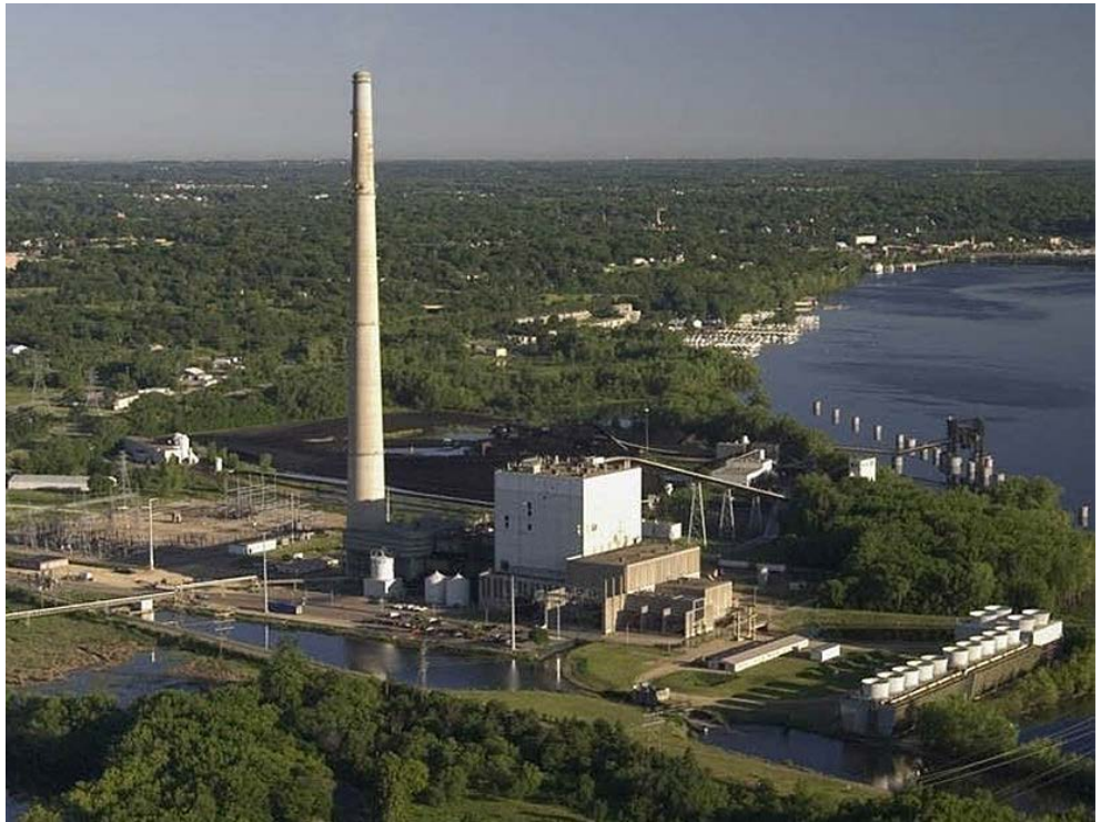
King Power Plant | Xcel Energy
